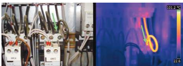
Thermal imaging analysis of a main switchboard. Real image on the left, thermal image on the right.
