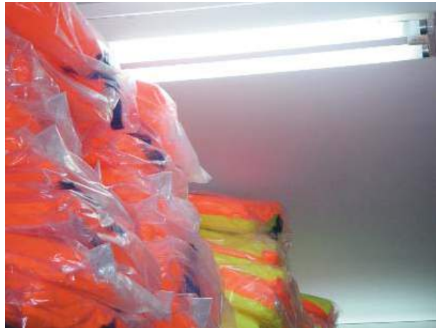
Plastic material stored near lighting
