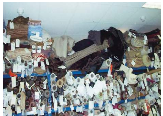
Obstructed automatic detectors
