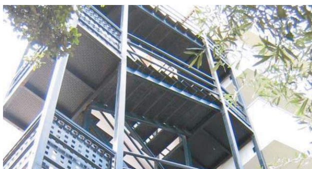
External emergency staircase
