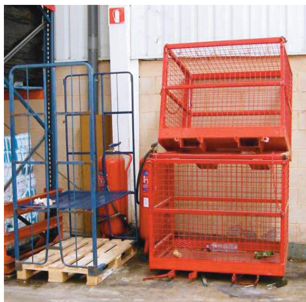
Extinguishers obstructed by loading equipment
